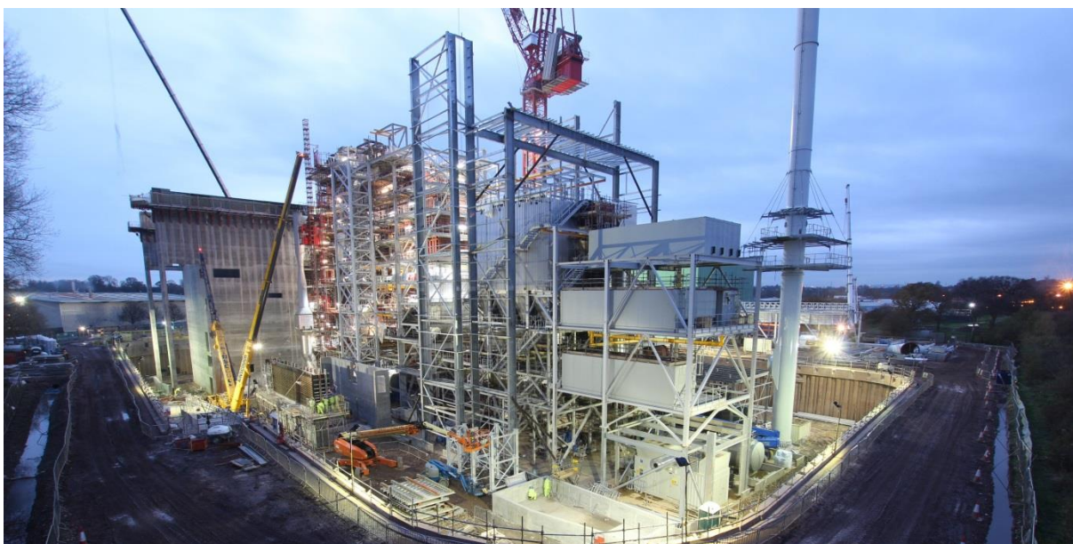
Envirecover Energy from Waste facility under construction.
